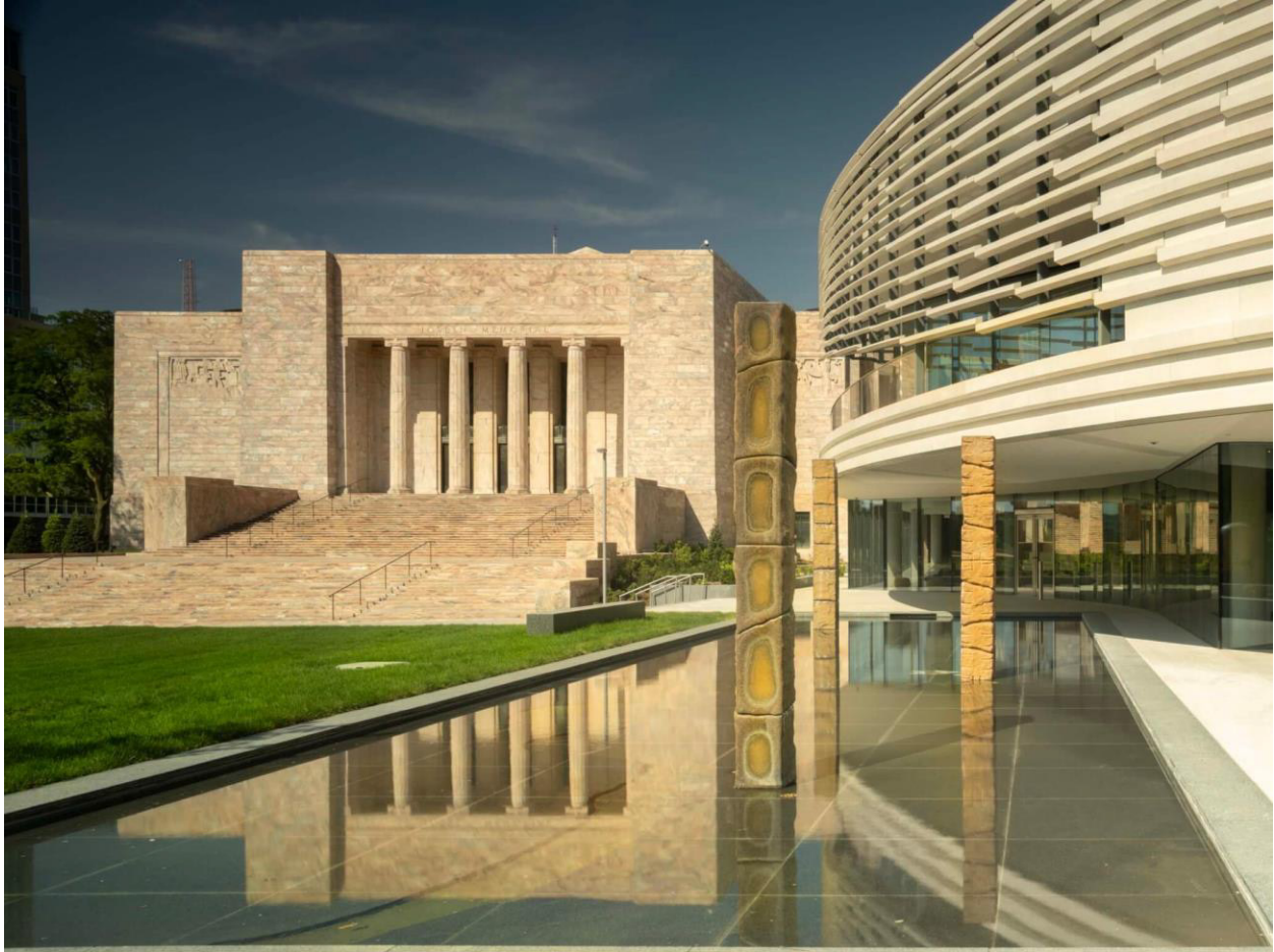
The rectilinear rigor of the original building softens into a contemporary curve. (Nic Lehoux)
