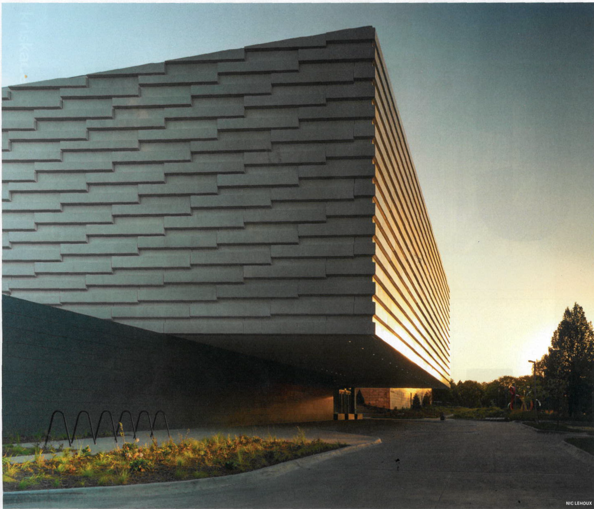
The new addition respects the rosy marble of the existing buildings but harmoniously updates the facade to reflect contemporary attitudes.
